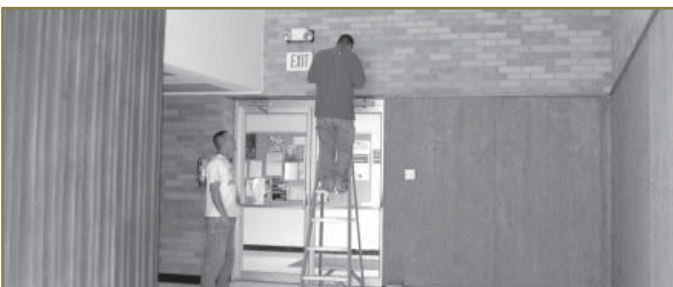
MAMPAC Workmen working on lobby renovations. Need outline
